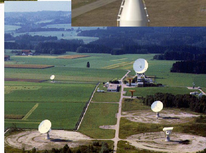
Weilheim Ground Station
